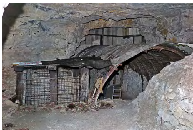
La Targette, upper level of tunnels looking back at shoring still in place
